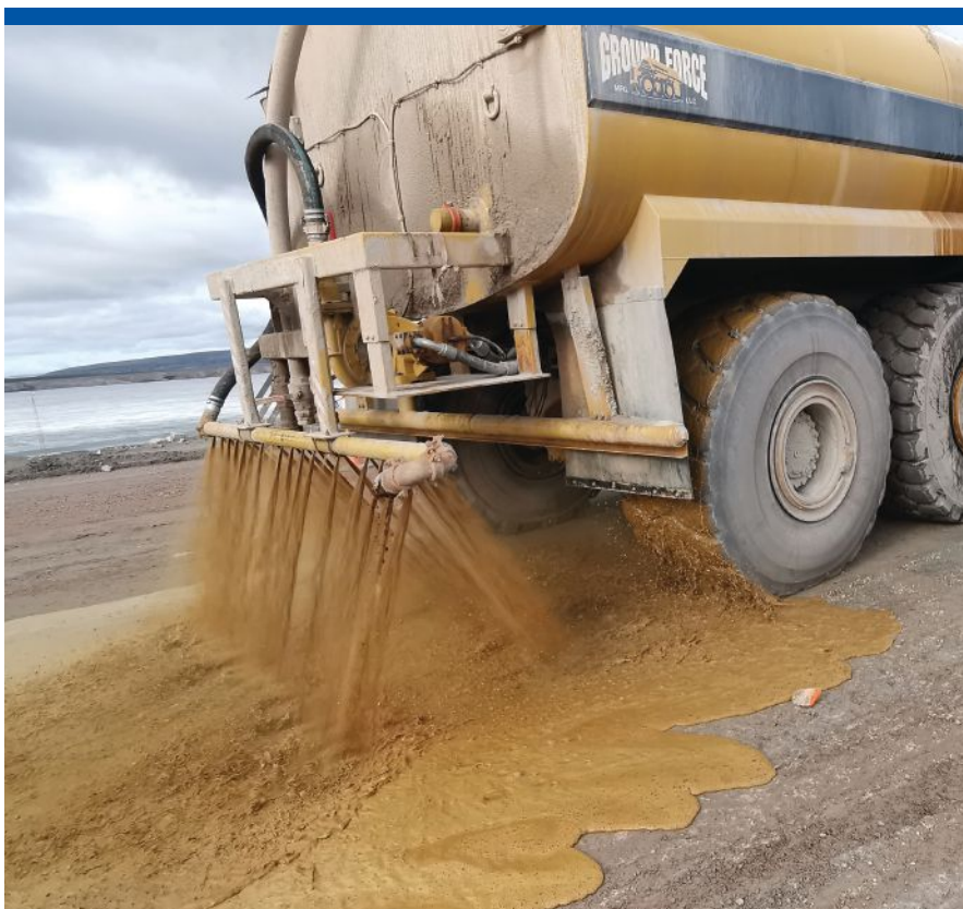
Applying DUST/BLOKR with a water truck. Photo: Baffinland.
